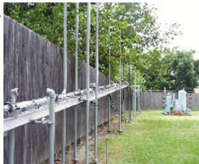
Hilly-Terrain Pipeline Test Section (Hill Configuration)
